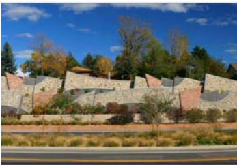
28th Street Soil Nail Wall
